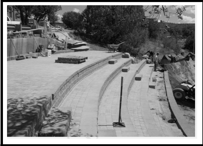
Wasted educational funds--the center field concrete plaza.
