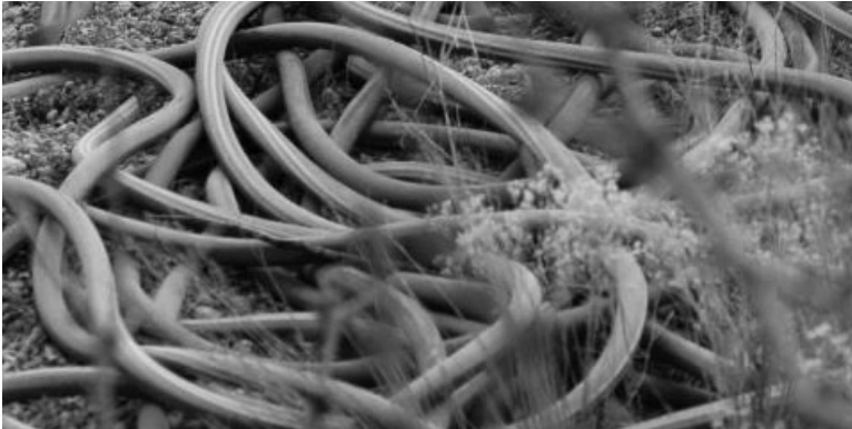
Decaying cracked hoses -- 2008
